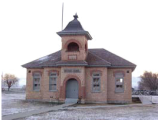
Fairfield School House, 1898
